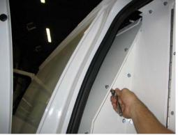
Begin to tighten <u>ALL</u> loose hardware on the remainder of the unit, being sure to align edges and bends of materials being tightened. This will square the unit to itself.
